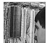
Easily mountable on standard 66 blocks, OnLine provides more complete and longer lasting protection than conventional communication line protectors.
